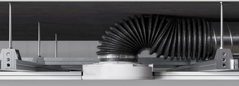
The vent connects to standard 100mm diameter ducting for use with an inline fan system. This makes it an idea choice for those looking for premium finishes.
